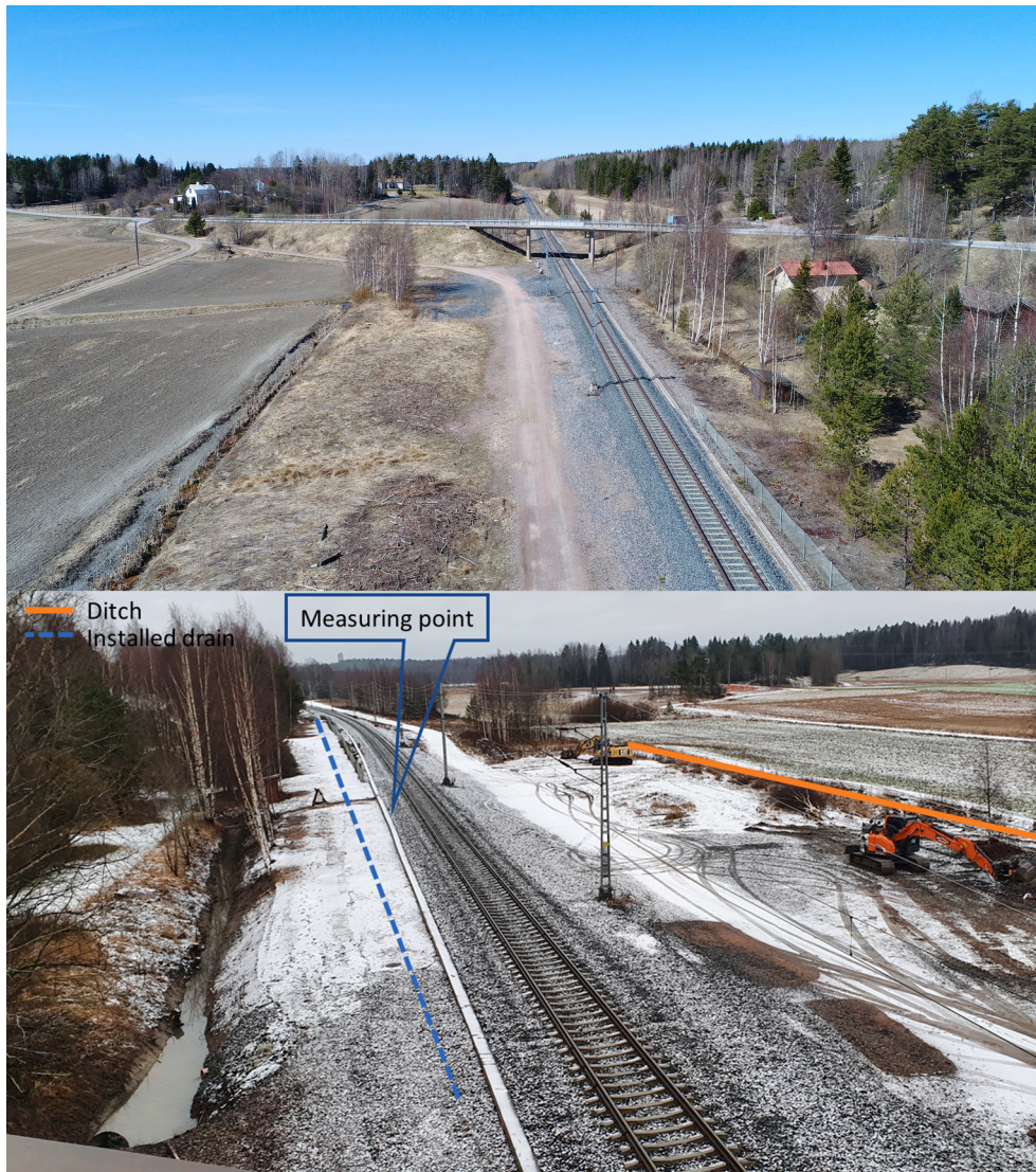
Fig. 2. The areal picture of Km 44 before and after the drainage improvement from opposite perspectives. The track is on flat terrain, and the drainage was not working properly. Photos taken on May 04, 2017, and January 29, 2020.
