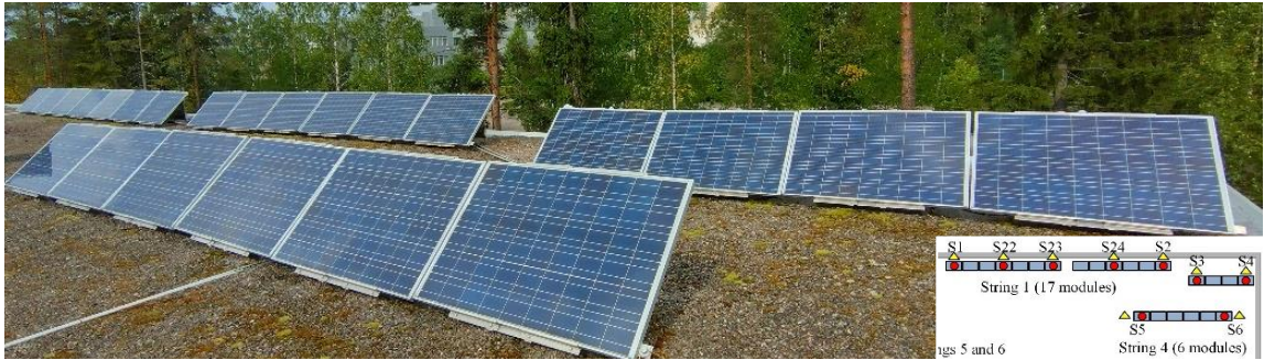
Figure 5.2.14. Picture and layout (down-right corner) of the 23 PV modules which the measured data is used in this thesis.
