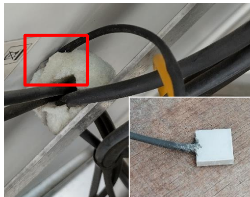
Figure 5.1.4. Pt-100 sensor inside of the aluminum sink (down-right) and the sink installed on back of the PV module (red box).
