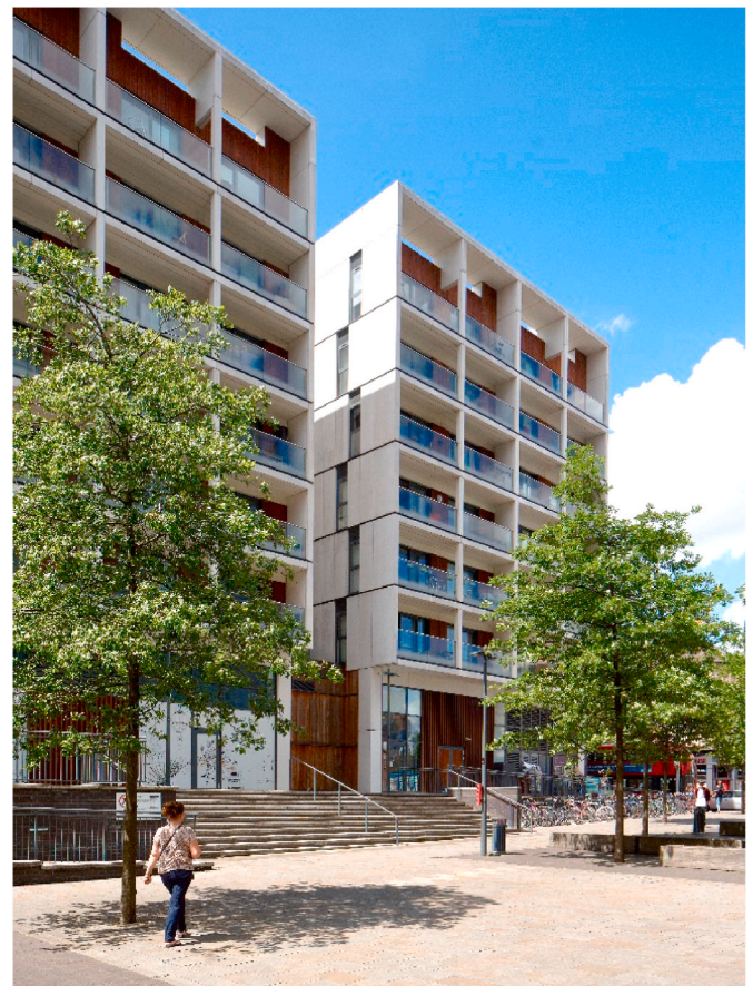
Fig. 4. Light coloured surfaces, planting, overhangs and side-fins, that shade glazing, mitigate overheating risk in these East-facing apartments. Architect: John McAslan + Partners. Photo: Joe Clark ( http://joelark.photo/ ).
