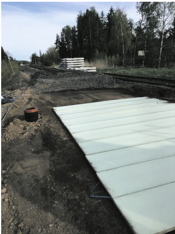
Figure 12. Frost insulation board installation in progress. Photo credit: Mikko Sauni.
