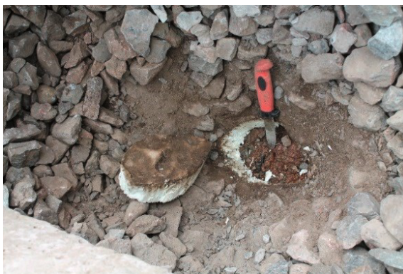
Fig. 5. A frost insulation board underneath ballast at sample point 216+068. Photo credit: Toni Saarikoski.
