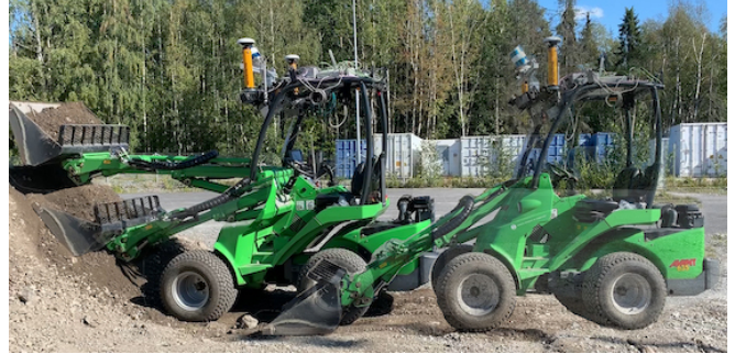
Fig. 1: Avant autonomous robotic wheel loader performing earth moving. Example videos in the supplementary material
