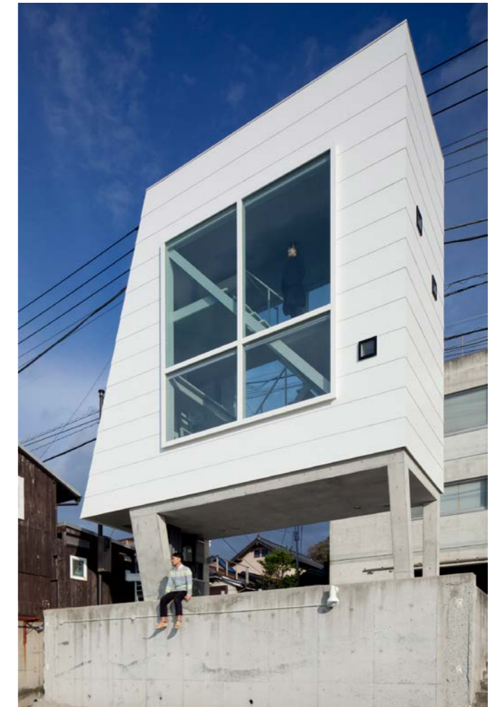
Yasutaka Yoshimura's Window House
