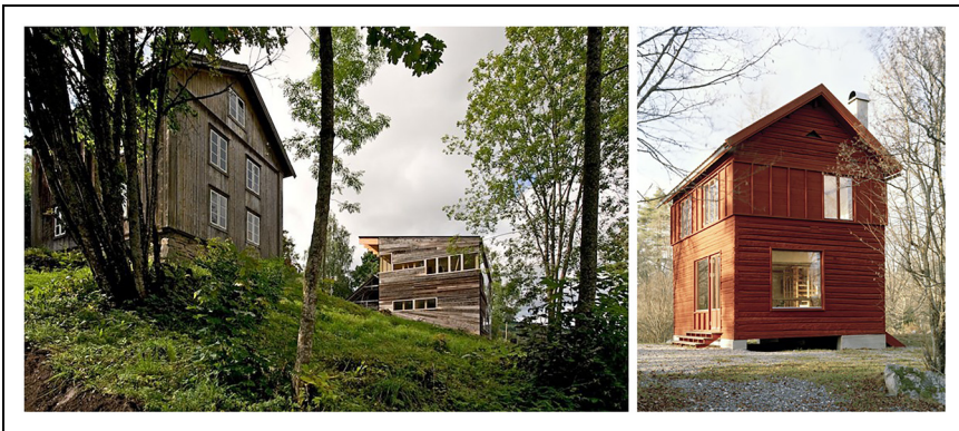
Figure 1. Vernacular barns re-interpreted. Farm House (left) Norway, where only claddings of the previously existed barn were used to cover the new barn-inspired house. Quite interestingly, the old main building is used only for guests and storage. © Jarmund/Vignæs AS Architects MNAL. Nannberga House (right) is a relocated barn converted to a house. © Mikael Olsson, General Architecture.
