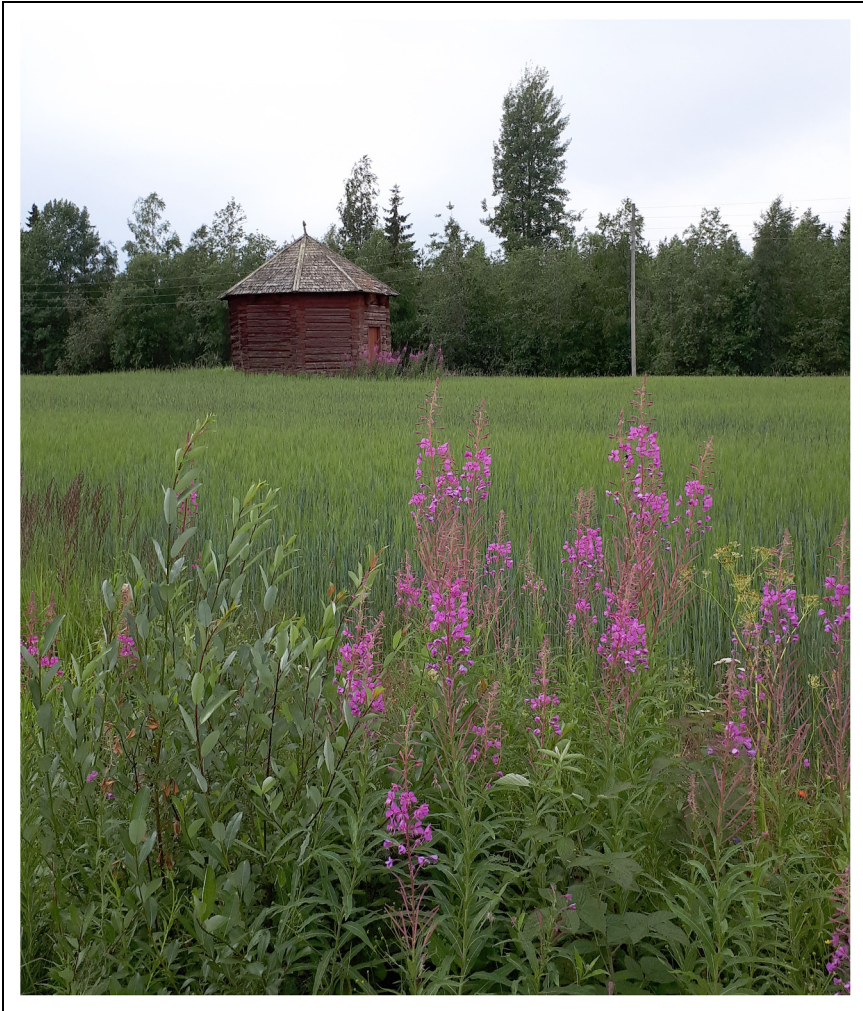
Figure 5. This small barn in Western Finland has an atypical hexagon-shaped floor plan, but typical setting as an accent of agrarian landscape. The beautifully weathered façade is painted with natural red ochre. Photograph © Iida Kalakoski
