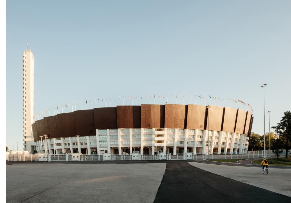
Helsinki Olympic Stadium from 2020 with its wood and concrete façade (Tuomas Uusheimo) [6]
