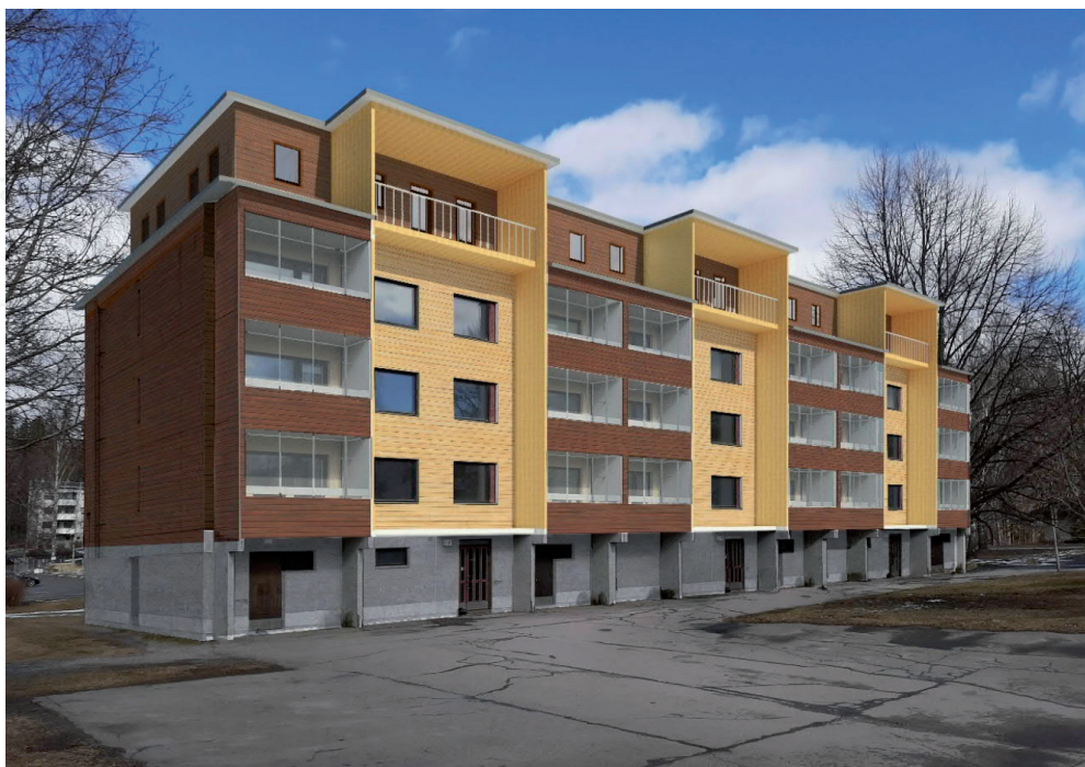
Figure 2. Representative image of wooden additional floor construction.
