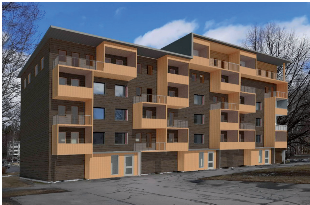
Figure 3. Representative image of wooden facade renovation.
