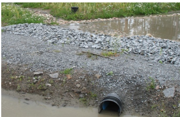
Figure 5 - Biofilter to manage stormwater in Tampere, Finland (City of Tampere, 2019)
