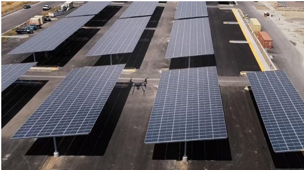
Figure 4.4. PV system inspection using drone with thermal camera [36].
