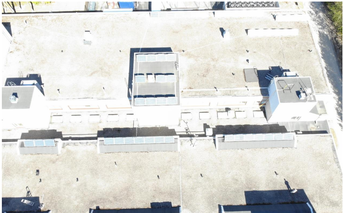
Figure 5.3. Aerial image for Part of Tampere University Solar PV power plant.
