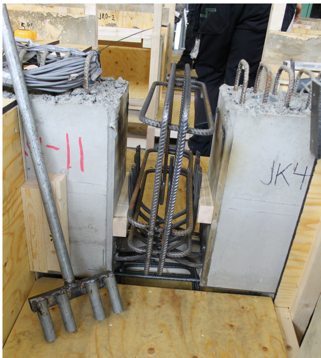
FIGURE 4 Diaphragm during reinforcement work, bent bottom strands and strand bending device
