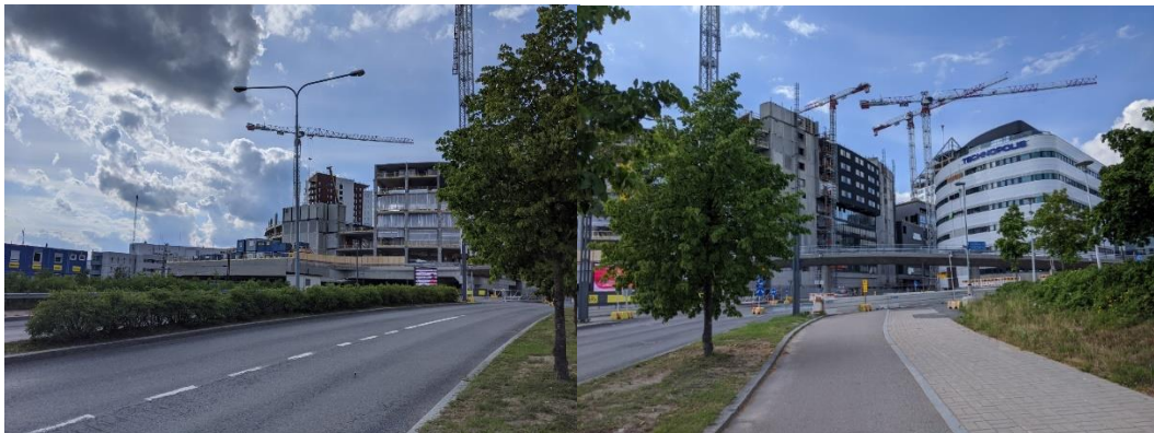
View from south of the arena construction site and the deck.
