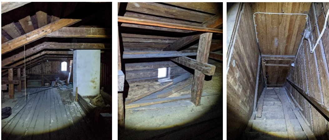
Attic space and the southern stairway.
