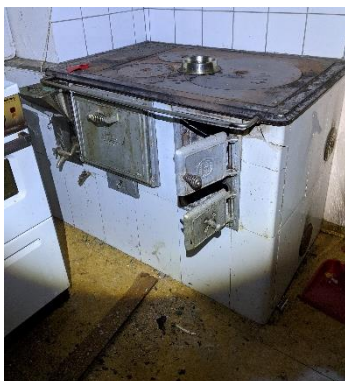
Existing masonry and tin fireplaces and kitchen stove.
