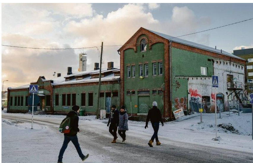
Tavara-asema, view from north-east. The footprint of the demolished warehouse is visible on the north façade. From Kansanuutiset, 11.1.2018
