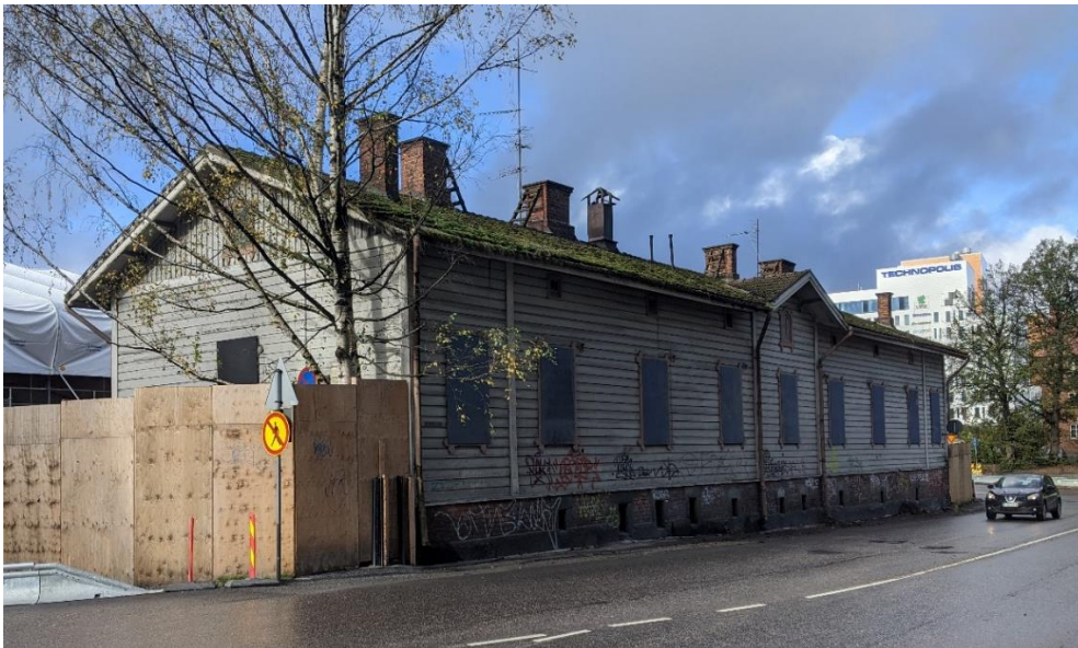
Tampere railyard's residential building, current status.
