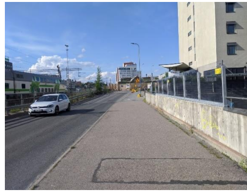
Unpleasant pedestrian path on the edge of the railway.
