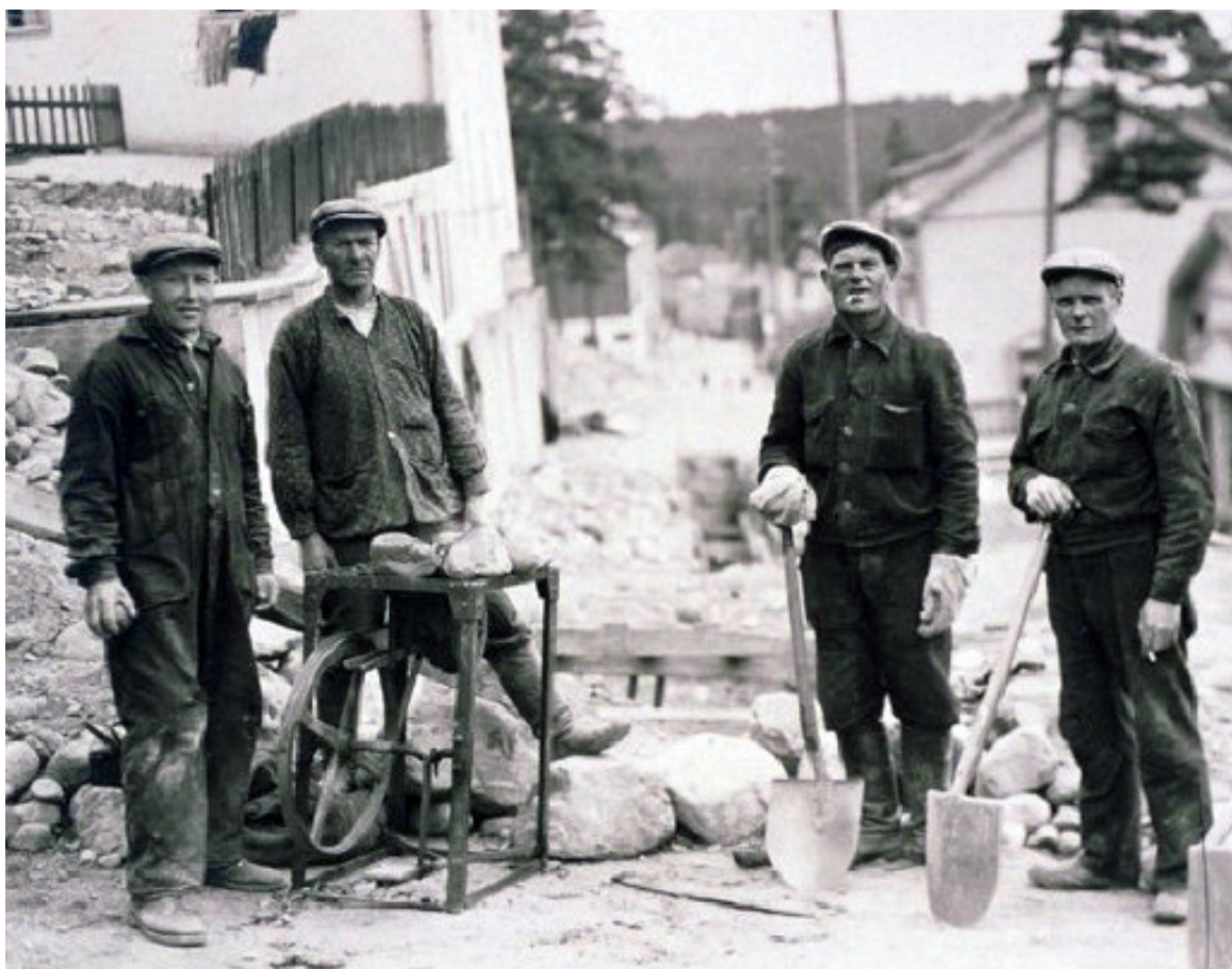
Picture N° 2. Installing the water mains.
