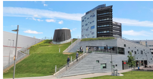
Figure 1. Photograph of the pilot building Kampusareena.
