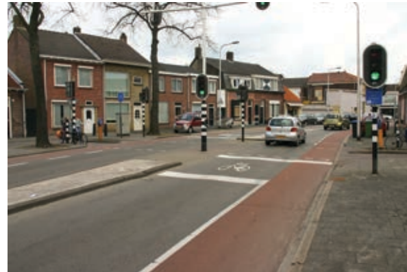
Figure 115. Advanced stop line for cyclists turning onto the intersecting cycleway. (Tilburg)
