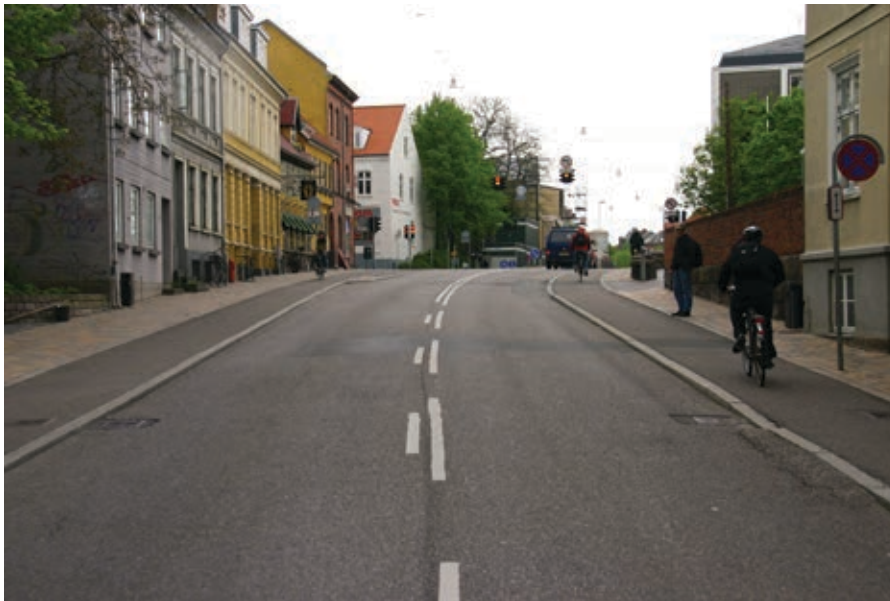
Figure 63. Sometimes it is necessary to designate part of the pavement for cyclists. Cycling and pedestrian safety can be increased by using distinctly different surface materials. One-way cycleways allow sufficient space for pedestrians on both sides of the street.
