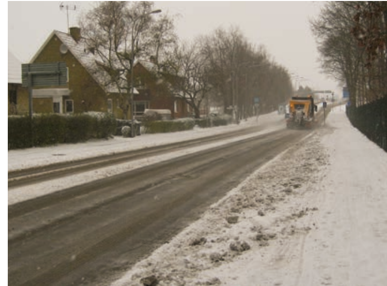
Fig. 3. The excess snow ploughed from the road often piles up on cycle paths and footways located next to the road.
