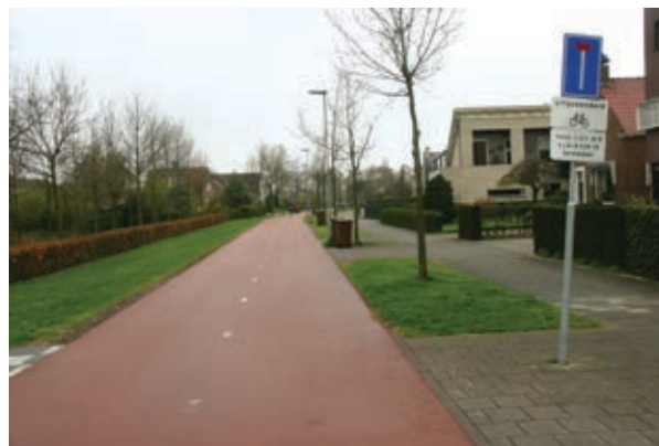
Figure 15. A high quality connection from the residential area to the centre. Cars can use the cycleway to access the driveways, but through traffic is prohibited. (Breda)
