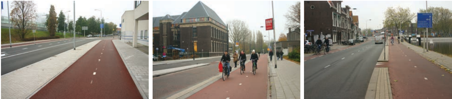
Figures 39, 40 and 41. One-way cycleways are usually the best option on central streets. Two-way cycleways can be used to enable turning around to travel in the opposite direction without unnecessary street crossings. If only one side of the street is developed, the two-way cycleway is a good solution (figure on the left). Likewise, if the route is mainly two-way and busy, short sections should not be converted into two one-way routes (figures in the middle and on the right). A one-way cycleway can, however, be used on the opposite side of the street.
