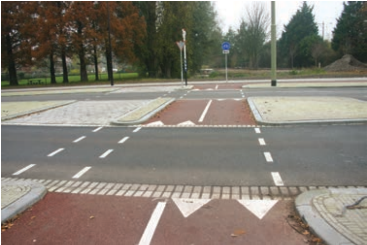
Figure 122. The cyclist's obligation to give way is also marked clearly on the islands. (The Hague)
