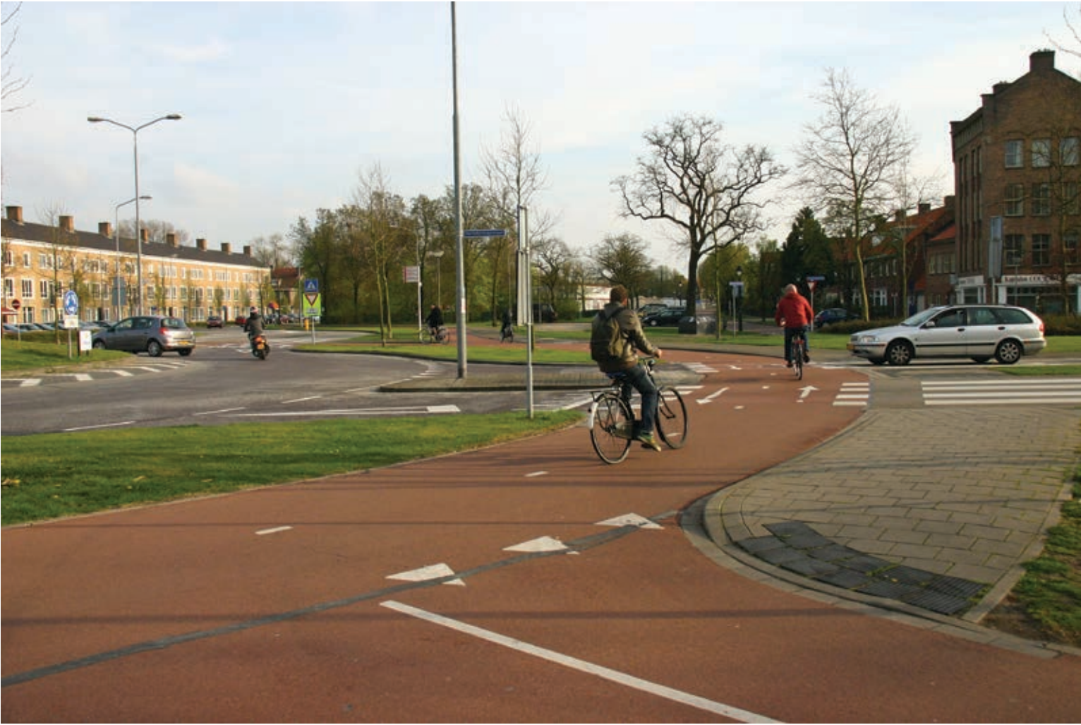
Figure 136. Smooth two-way cycling on a roundabout made possible through good designing. Good visibility distances and clearly marked cycling directions facilitate navigation on the roundabout and improve the safety of the cyclists. (s-Hertogenbosch)
