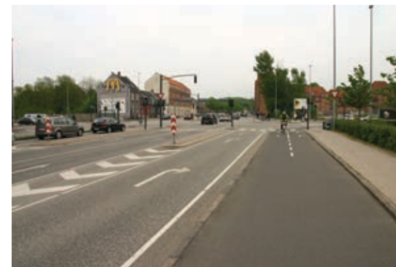
Figure 67. Due to the busy bicycle traffic on the street, the cycle lane takes up more space from the street surface than the roadway. The wider the lane, the safer it is for cyclists. (Odense)
