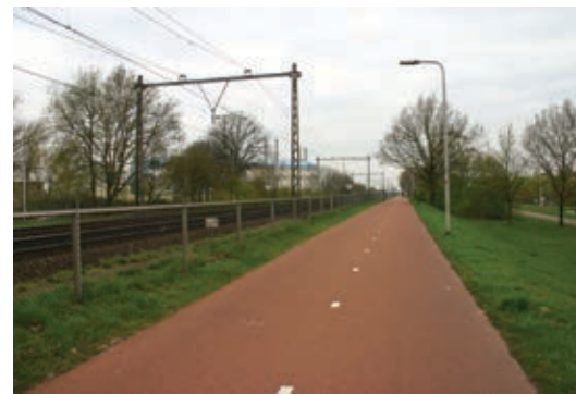
Figure 30. The flat ground next to railway tracks often provides an excellent location to build a cycle super highway. (Nijmegen)
