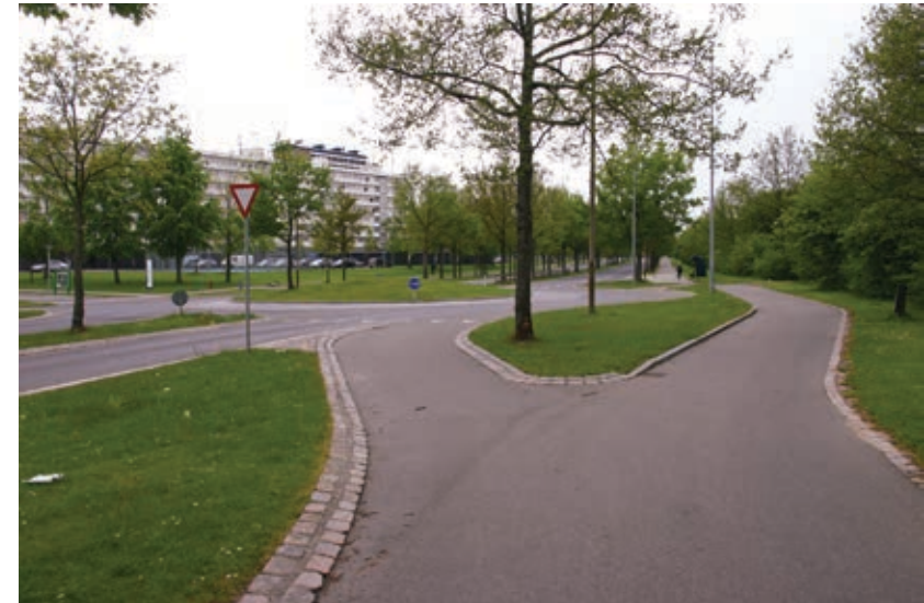
Figure 135. Straight cycleway bypassing a roundabout. Cyclist turning left use the roundabout. When on the roundabout, cars and cyclists share the same roadway. (Odense)
