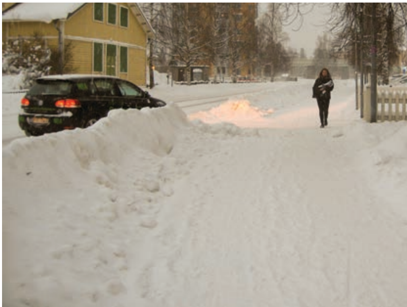
Fig. 14. The City of Umeå has opted to build green areas between the cycle paths and footways and the road, and use them for snow storage.
