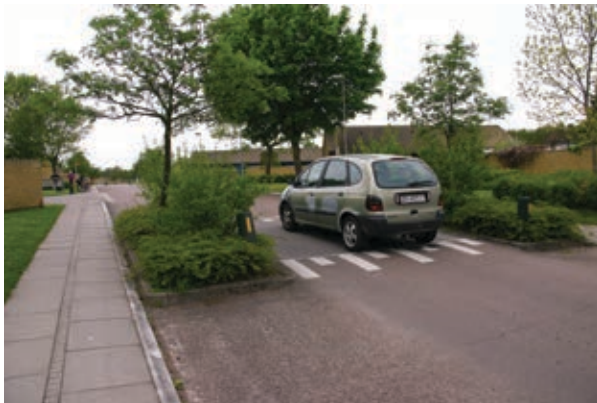
Figure 90. Planting can be used as traffic calming devices, adding simultaneously to the comfort of the street space. (Odense)
