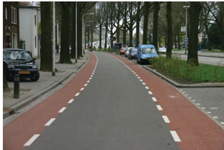
Figure 73. Colour can be used to make the advisory cycle lanes easier to notice. (Tilburg)
