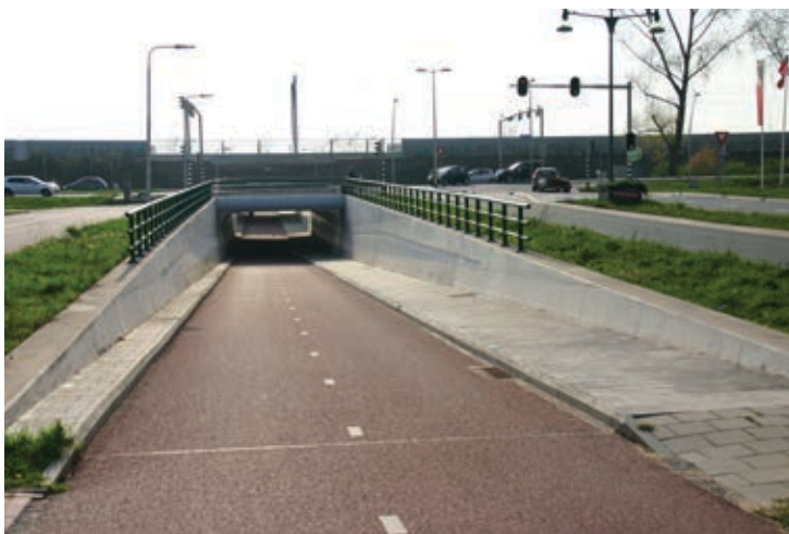
Figure 129. In this Nijmegen cycleway underpass, the steepness of the slope has been minimised (max 4%) by building a long ramp to the underpass and by raising the roadway (0.8 m). Pedestrians have a separate route in the underpass under the roadway.
