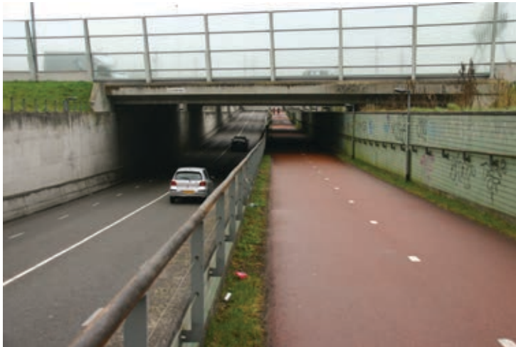
Figure 128. The slope to the cycleway underpass is not as steep as that to the roadway. There is no need for the cycleway underpass to be as high as the roadway underpass.
