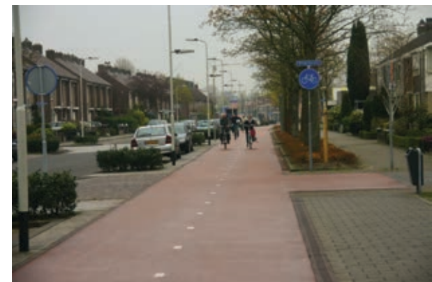
Figure 16. An example of street space allocation in a residential area. Different transport modes are separated, with the emphasis on the cycleway. The four-metre wide route is straight and fast. (Breda)
