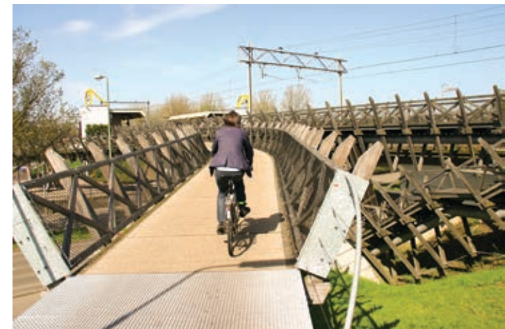
Figure 34. This combined cycling and pedestrian bridge in 's-Hertogenbosch has been built in a style similar to the railway bridge next to it.
