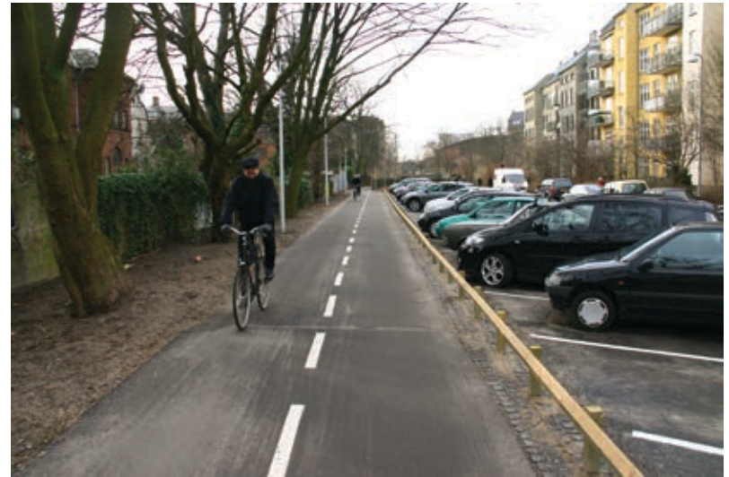
Figure 18. A rail is an excellent solution where space is limited. A good quality cycleway can be built on a fairly narrow strip. (Copenhagen)
