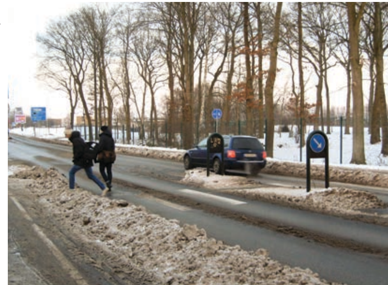
Fig. 4. In winter maintenance, intersections are often problematic. The snow tends to pile up at the ends of the pedestrian crossings, making them more difficult to use for pedestrians and cyclists.
