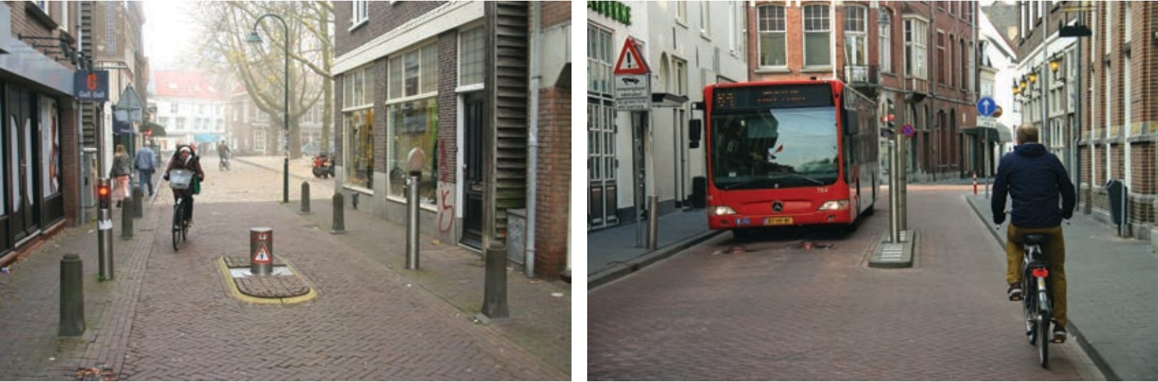
Figures 104 and 105. Delft (left) and 's-Hertogenbosch (right) use automatic bollards to restrict access by cars to the city core. Cyclists can bypass the island with ease. The bollards are equipped with thermostwitch-controlled heating to ensure proper operation in cold conditions.
