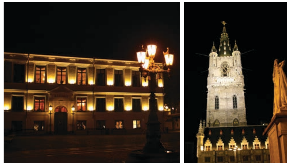
Fig. 23. Lit frontages can be used to emphasise important buildings and to illuminate the environment effectively. (Lund, Gent)
