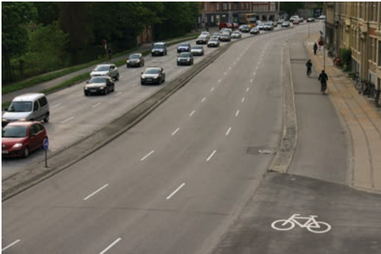
Figures 51 and 52. If the traffic flow increases, the cycleway should be separated from the vehicular traffic with a separator lane. (Copenhagen)
