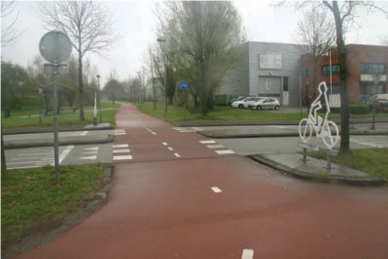
Figures 119 and 120. A cycling highway crosses a collector street. Motorists give way to the cyclists.
