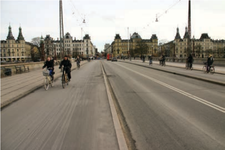
Figures 44 and 45. In Copenhagen, split kerb stones are often used to separate general traffic streets from the one-way cycleways. Split kerb stones are also used to separate the pavement from the cycleway. Due to the daily flow of approximately 40,000 cyclists on Nørrebrogade (figure above), the one-way cycleways are four metres wide on both sides of the street.
