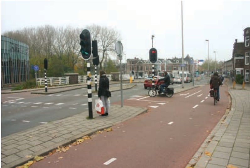
Figure 123. At intersections, cyclists adhere to similar rules to vehicular traffic. Markings for getting into the correct lane and the obligation to give way are clear. Pedestrians use the pedestrian crossing. (Delft)
