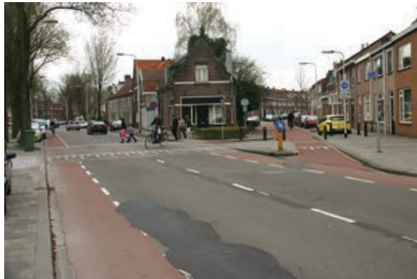
Figure 114. Cars are not allowed to turn on the bicycle boulevard diverging to the right. The island is there for the cyclist coming from the bicycle boulevard. (Tilburg)
