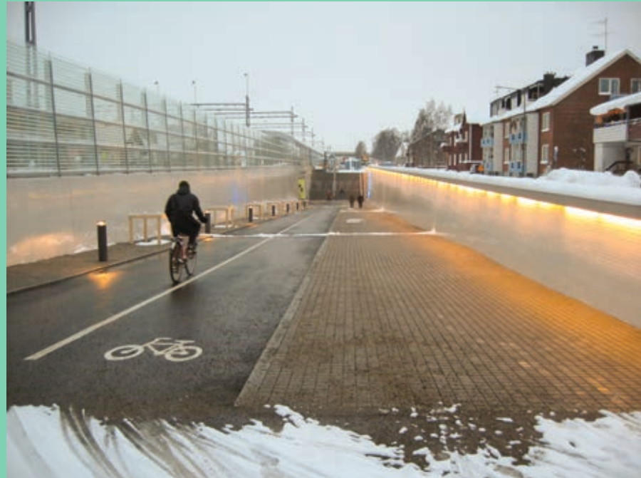
Fig. 34. In Umeå, some underpasses, like the one leading to the railway station, are heated. Lighting is also carefully designed.
