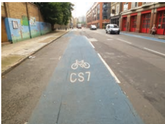
Figure 68. Contrary to the figure, cycle lanes should be straight with no curves to accommodate on-street parking.
