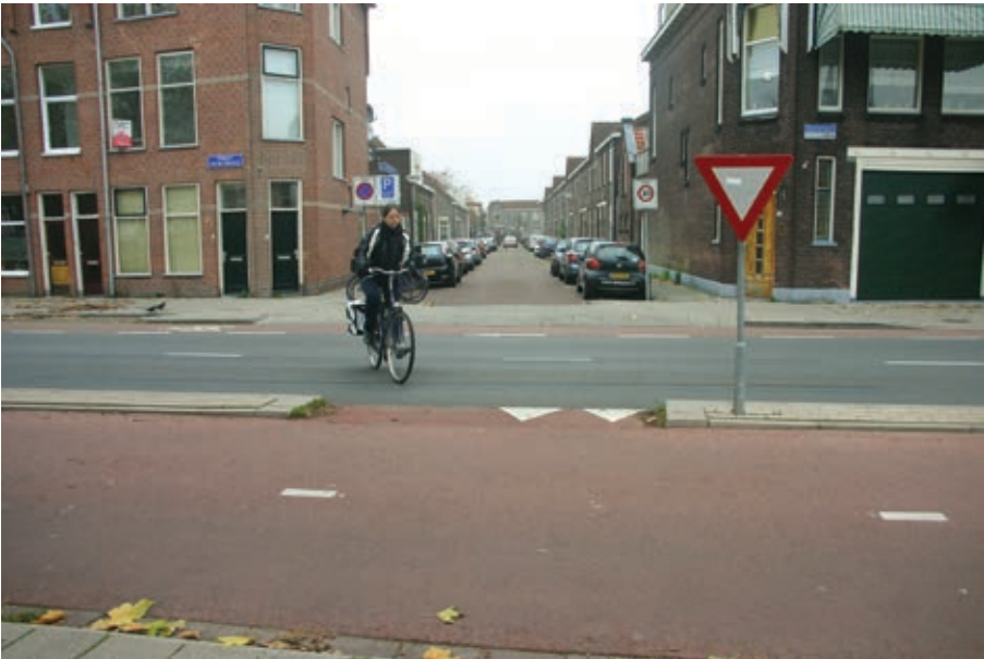
Figure 126. Cyclists coming from the side street have straightforward and clear access to the cycleway. When crossing the main street to turn to the side street, cyclists must give way to the vehicular traffic. (Delft)
