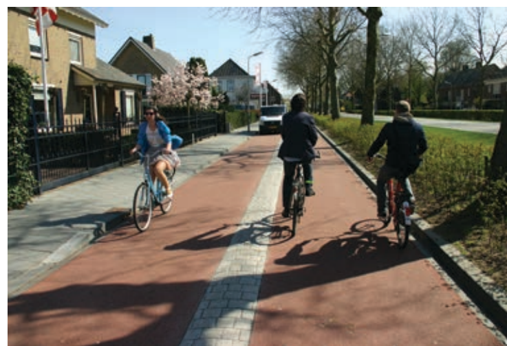
Figures 76 and 77. This access lane in 's-Hertogenbosch has been converted into a bicycle boulevard.
