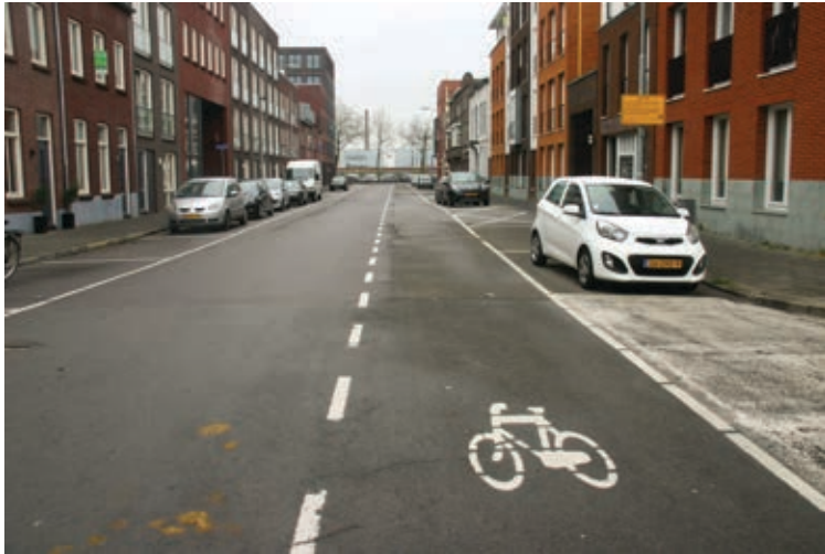
Figure 95. To improve safety, advisory cycle lanes can be used on one-way streets, permitting cycling against the traffic. (Breda)
