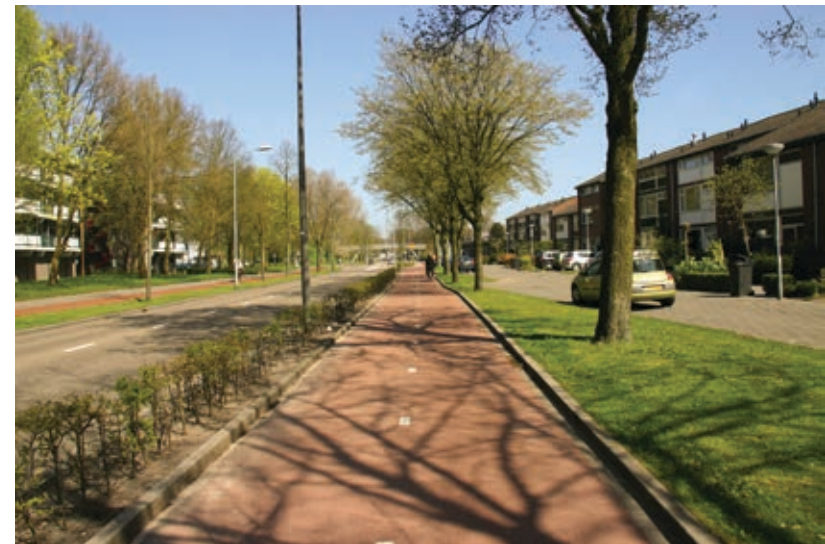
Figure 43. In 's-Hertogenbosch, a one-way cycleway was converted into this two-way cycleway so that children do not need to cross the road on their way to school. The cycleway gets narrower further down the route to allow space for the trees.
