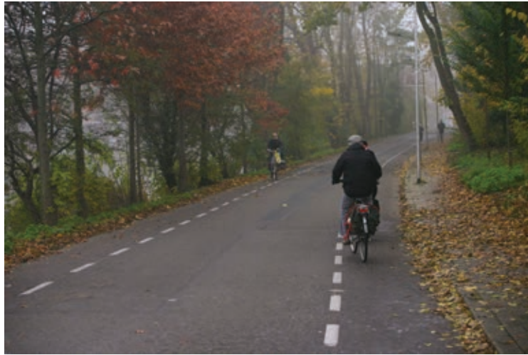
Figure 71. The Netherlands have advisory cycle lanes for cyclists. Cars are allowed to use the lanes in order to avoid oncoming traffic. Advisory cycle lanes are used when the street is too narrow for cycle lanes, but cyclists nevertheless need a designated space due to busy car traffic or high driving speeds.
