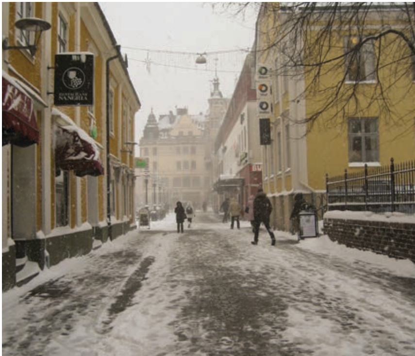
Fig. 9. In Linköping, the heating system keeps the pedestrian areas clear of ice.
