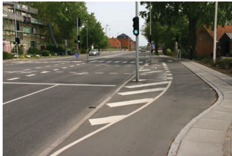
Figure 125. A cycleway intersection alongside general traffic streets. The intersecting streets have one-way cycleways. Cyclists coming from the left must give way to the cyclists going straight ahead. Those turning left have a separate lane. (Odense)
