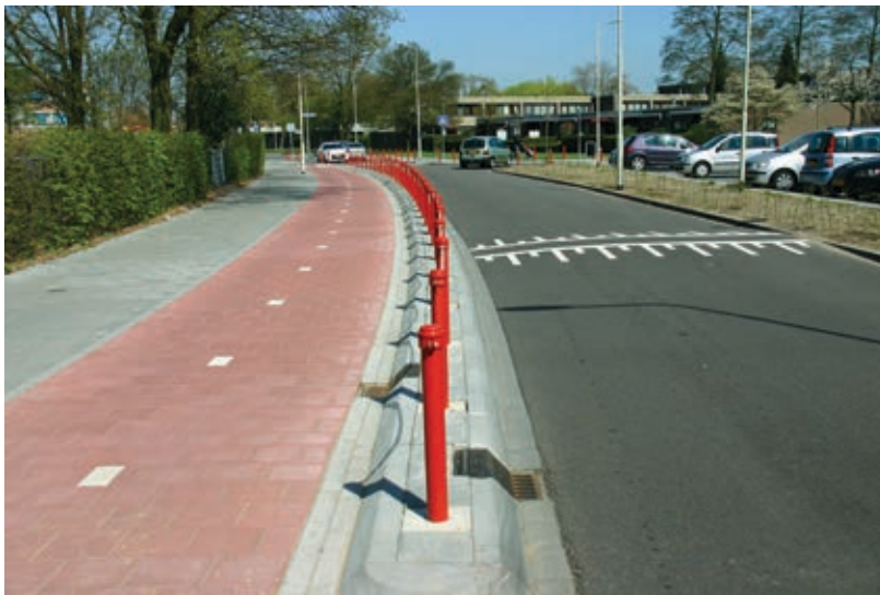
Figure 42. A section of the roadway has been separated to create a two-way cycleway. The structural barrier made of kerb stones, bollards and chains protects the children on their school journeys. Pedestrians and cyclists have separate lanes.
