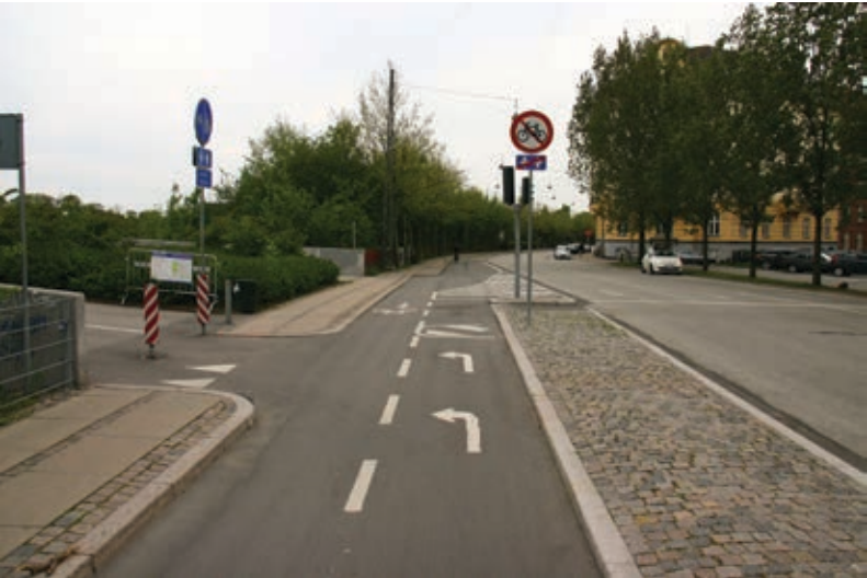
Figure 38. The point where the two-way cycleway becomes a one-way cycleway should have clear street markings. (Copenhagen)
