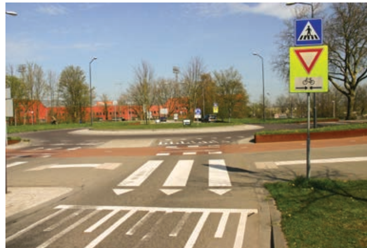
Figure 139. The obligation to give way to cyclists already on the roundabout is marked clearly. The guidance and warning surface for people with visual impairments is applied on the cycleway crossing. ('s-Hertogenbosch)
