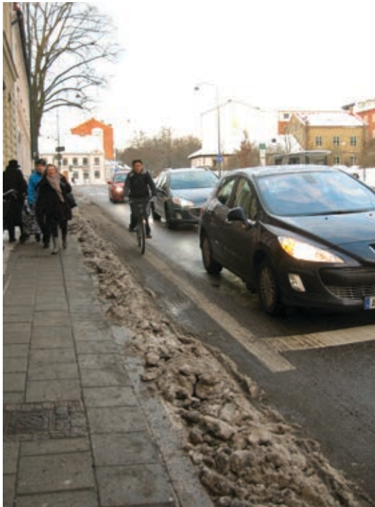
Fig. 2. Snow ploughed on cycle path makes safe movement difficult and encourages cyclists to use the road instead.
