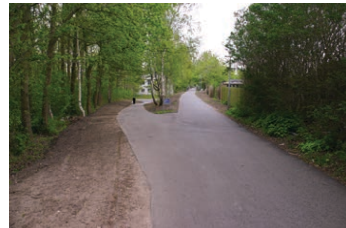
Figures 130 and 131. Grade-separated cycleway intersection. The ramp on the left leads down to an intersecting cycleway. The gentle slope increases cycling comfort. Signs are used as per regular road traffic. (Odense)
