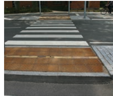
Fig. 21. Tactile paving indicating the beginning and end of the crossing. The distinctive colour helps to perceive the paving. (Odense)
