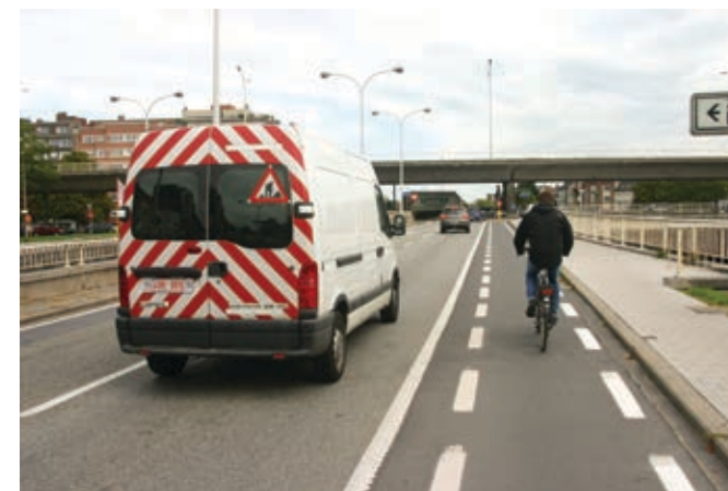
Figure 70. On busy streets with heavy traffic, a one-way cycleway is safer than a cycle lane. The safety of a cycle lane can be increased by making it sufficiently wide and using street markings to create a safety zone for the cyclists. (Ghent)
