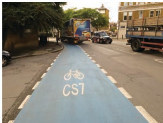
Figure 69. The cycle lane in the figure is not safe because heavy vehicles use it as a short cut.
