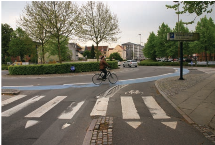
Figure 133. A one-way cycleway joins a roundabout next to a roadway. The barrier between the roadway and the cycleway prevents the motorists from using the cycleway as a short cut. (Odense)
