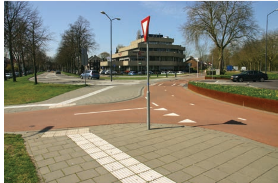
Figure 138. The cycleway encircling the roundabout has been raised above the level of the roadway. Two-way traffic is indicated with clear street markings and traffic signs. The motorist's obligation to give way is also clearly indicated. ('s-Hertogenbosch)
