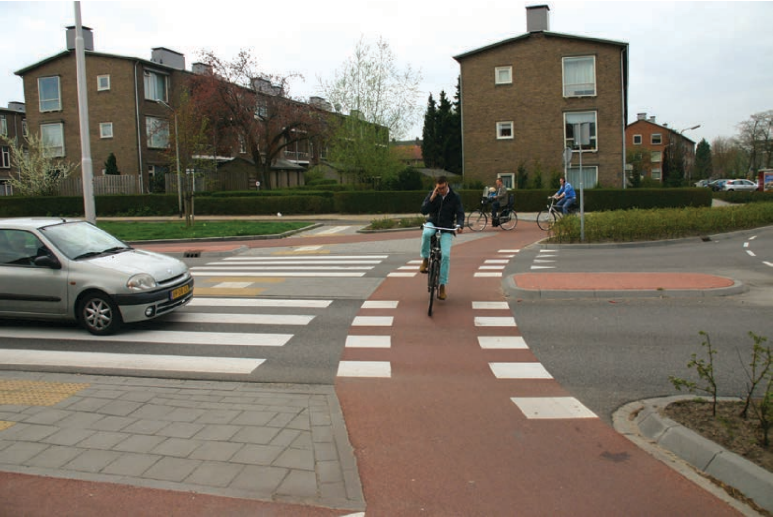
Figure 132. A separate one-way cycleway has been found to be the safest solution on roundabouts. (Nijmegen)
