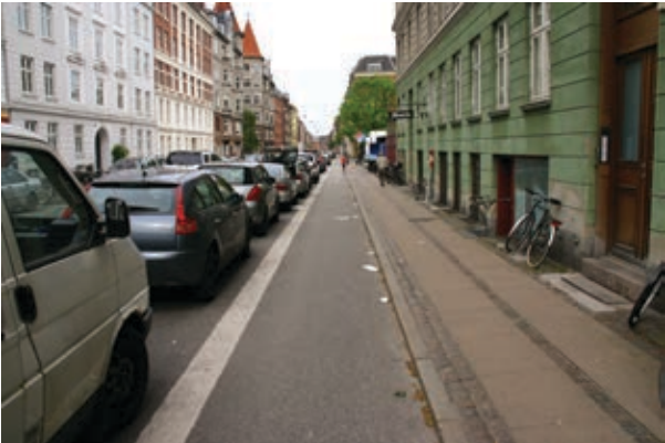
Figure 53. A one-way cycleway behind a row of parked cars on the street. The cycleway runs unobstructed alongside the on-street parking. (figures: left from Copenhagen, right from Odense).
