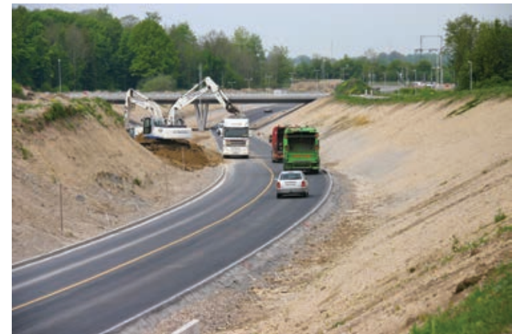
Figure 107. Construction work on the ring road around Odense city centre in 2012. The aim was to limit vehicular traffic through the centre. To avoid differences in levels, the cycleway runs along the cut.
