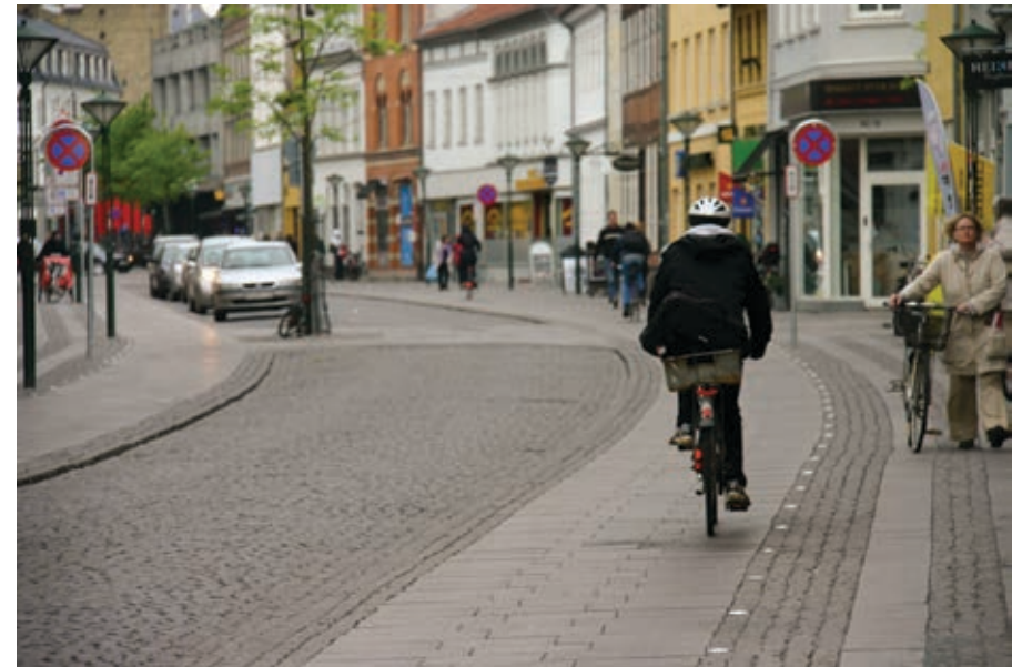
Figure 64. On Overgade in Odense, mixed traffic could be a safe option. For cycling comfort, however, designated cycleways separated by smoother surface material than the historical cobblestone surface of the rest of the street is a good solution – especially due to the busy cyclist flow on the street.
