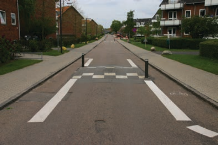
Figures 86 and 87. Cycling comfort can be increased by applying traffic calming devices for vehicular traffic only. Cyclists can bypass the devices. The cycle lanes in figure on the left are of the advisory cycle lane type. (Delft and Copenhagen)
