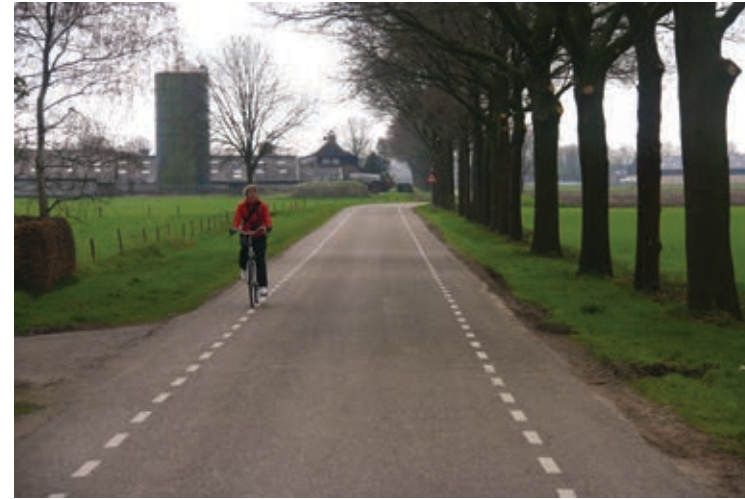
Figure 72. In the Netherlands, advisory cycle lanes are also used on the roads. Designated space helps to decrease the feeling of insecurity experienced by the cyclist due to heavy farm-bound traffic, for example. (Rijen)
