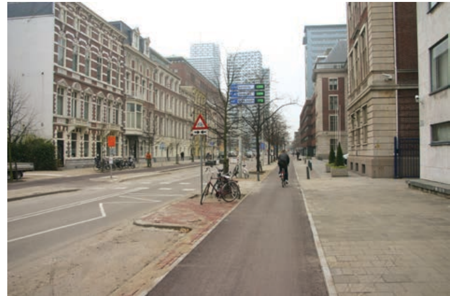
Figure 48. The roadway was made narrower to allow sufficient space for the one-way cycleways on both sides the street. The pavements are also wide enough. (The Hague)
