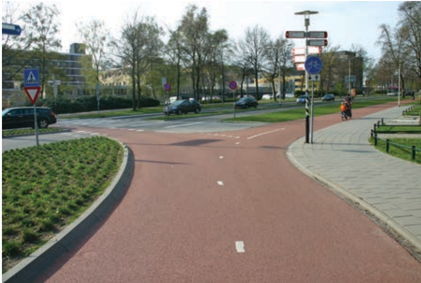
Figure 137. A two-way roundabout cycleway changes into a one-way cycleway. Due to the high cyclist flows to and from the university, parts of the roundabout cycleways have two-way traffic. Good design ensures that the solution works properly. (Nijmegen)
