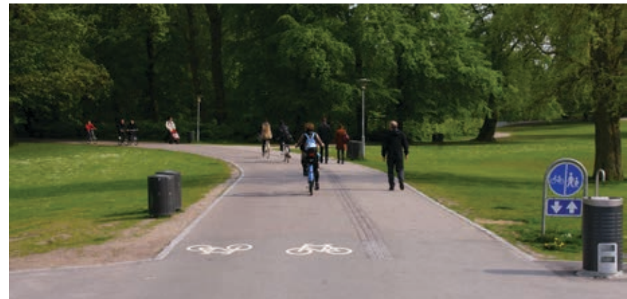
Fig. 19. On an accessible pedestrian and cycle path, the pedestrians and cyclists are clearly segregated. The surface is smooth, and there is enough room for wheelchairs and pushchairs. (Odense)
