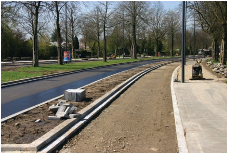
Figure 47. An example of a high quality one-way cycleway: the other lane of the roadway is converted into a one-way cycleway with a structural barrier separating it from the roadway. (s-Hertogenbosch)
