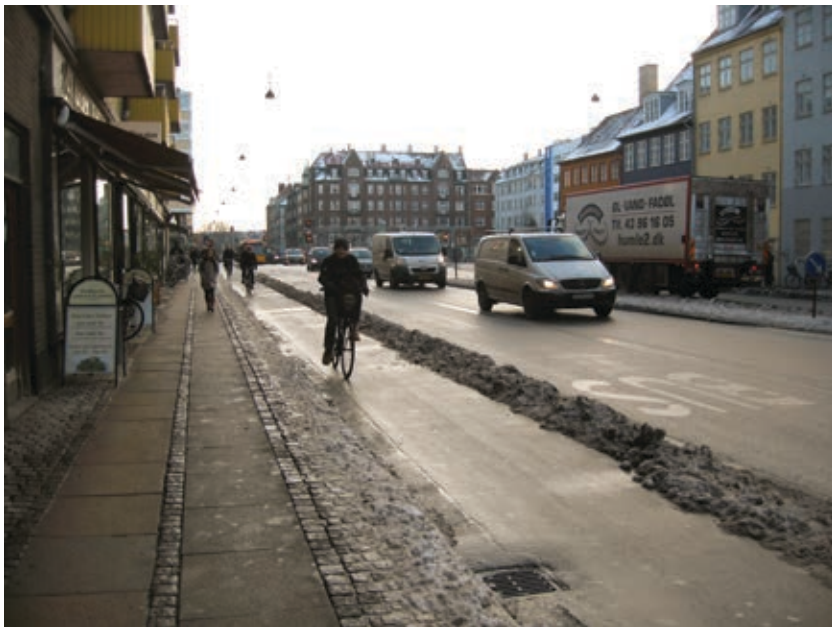
Fig. 24. In Copenhagen, planners have added a half-metre wide space for snow between the cycle path and road, eliminating the need to transport snow during a normal winter.
