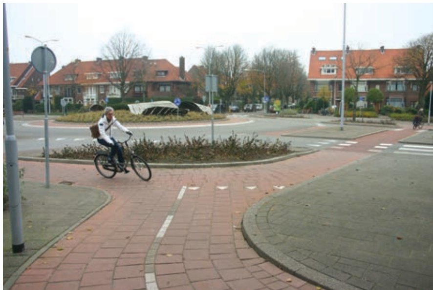
Figure 134. A two-way cycleway joining a one-way cycleway on a roundabout. The solution works. It is similar to the one used by the cars on the roundabout. (The Hague)
