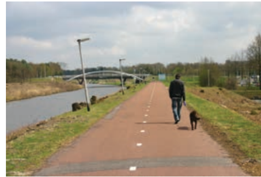
Figure 28. Cycleway running along the river bank from Tilburg to the east toward the city of Breda. Due to the low number of pedestrians, they are allowed to use the cycleway, eliminating the need for a separate pedestrian path.
