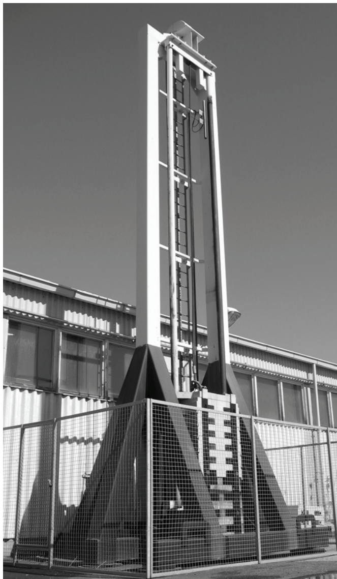
Fig 5. The bundle rack, height about 9 metres.
