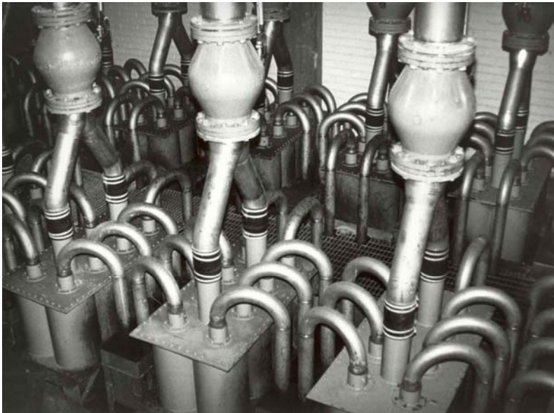
Figure 5. Multistage pressure swirl concentrators specially designed by Seppo Ryyänen for Pätt wastewater treatment plant. They were in operation from 1985 to 2001. (Häkkinen et al 1987)
