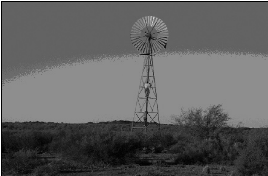
Illustration 3. A typical wind turbine in the Northwestern Cape, South Africa, on the farm Nanibeas, Brandvlei District. The wind turbine, also known as a windpump in South Africa, was manufactured in the industrial city of Vereeniging in the mid-twentieth. After having fallen into disuse it was recently restored, with good effect by the owner of the farm, Mr. Francis Visagie. (Photograph: Magda Morrison (2003) with additional information by Theo Venter), Editor.
