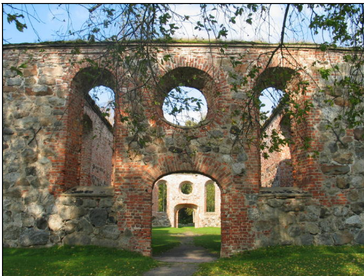
Figure 3. Ruins of old Vaasa after the Great Fire of 1852 (Photo: T. Katko).
