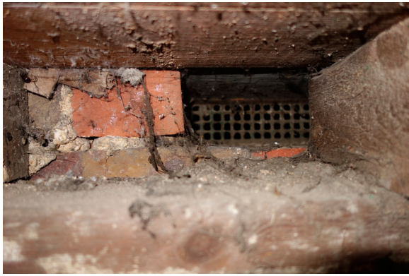
Figure 2. An airbrick in between the joists.
