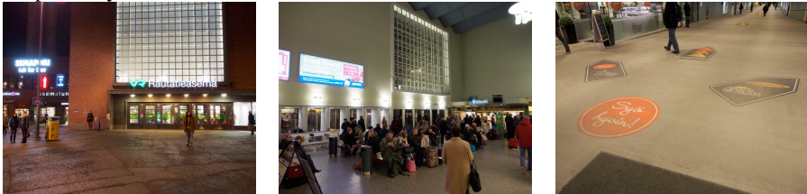
Fig. 1. Left: Tampere Railway Station picture from the City Centrum direction showing the main façade. Middle: Waiting hall of the railway station has large wall areas, mainly populated by static advertisements. Right: Signage on the railway station mostly advertises the stores on the building.
