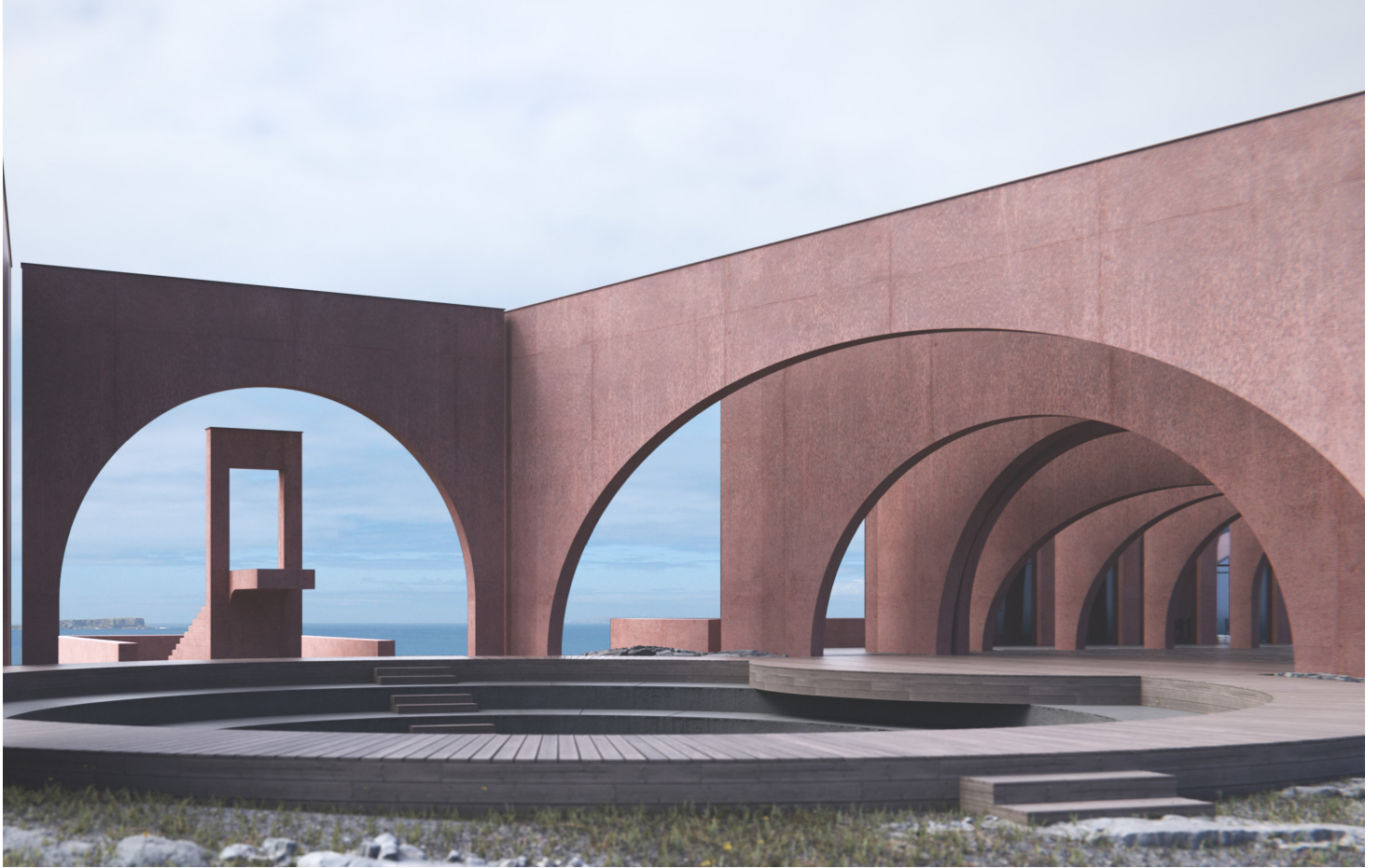
Outdoor stage combined with multiple types of staging
