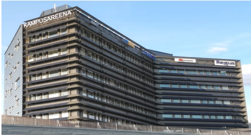
Figure 4. Darker walls that are facing south-east, west and south-west shows solar panels on the building [18].
