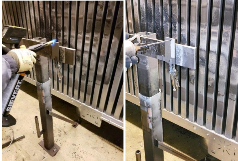
Figure 24 Pre-heating and spraying (low pressure).
