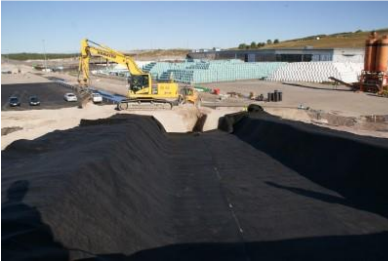
DCS04318 Kaivanto putkille (22.8.2019)
