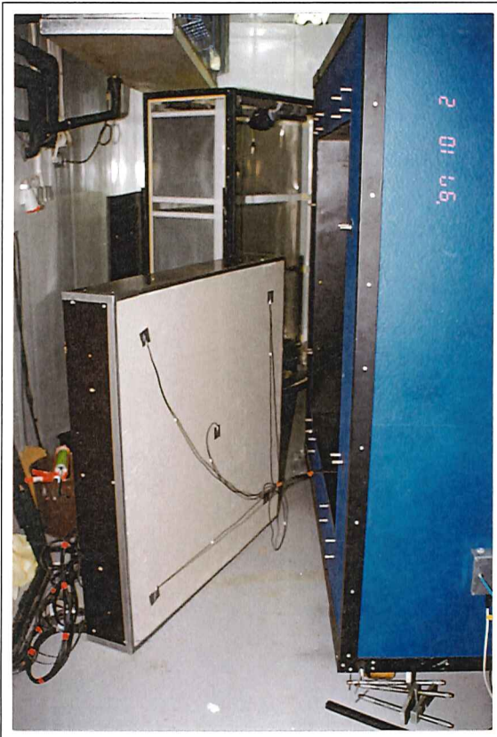
III 1. Surface temperature sensors were installed on the internal surface of finished test wall. Subsequently, the wall was ready for installation in the test opening.
