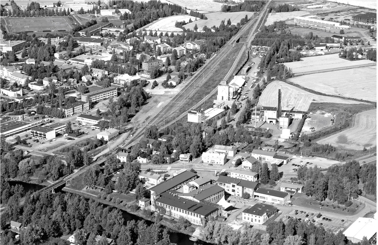
Figure 1. Old Paukku seen from south. The centre of Lapua on the left.
