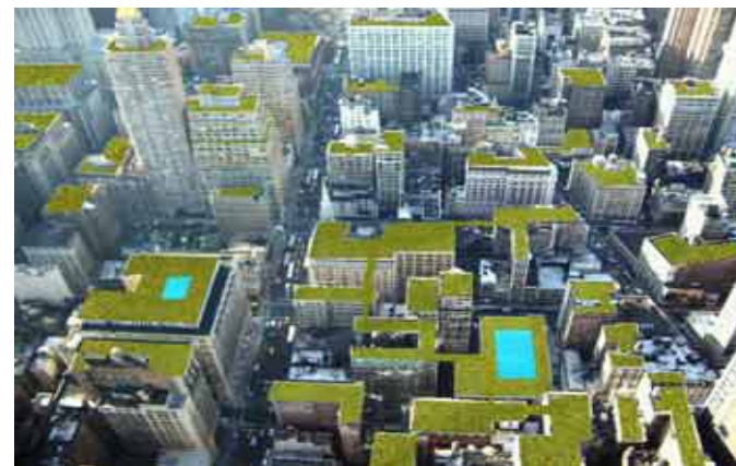
Figure 5: Green roof assumed to be suitable for 3/4 of the total roof area.
