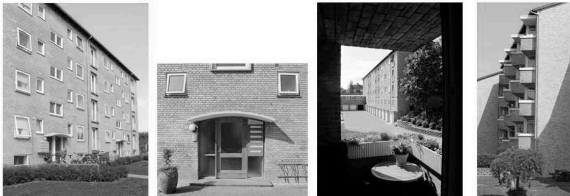
Figure 1: Typical housing block, entrance, balconies
