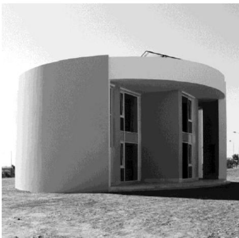
Figure 3.1: as built case - energy-efficient construction method of the GUTech EcoHaus
