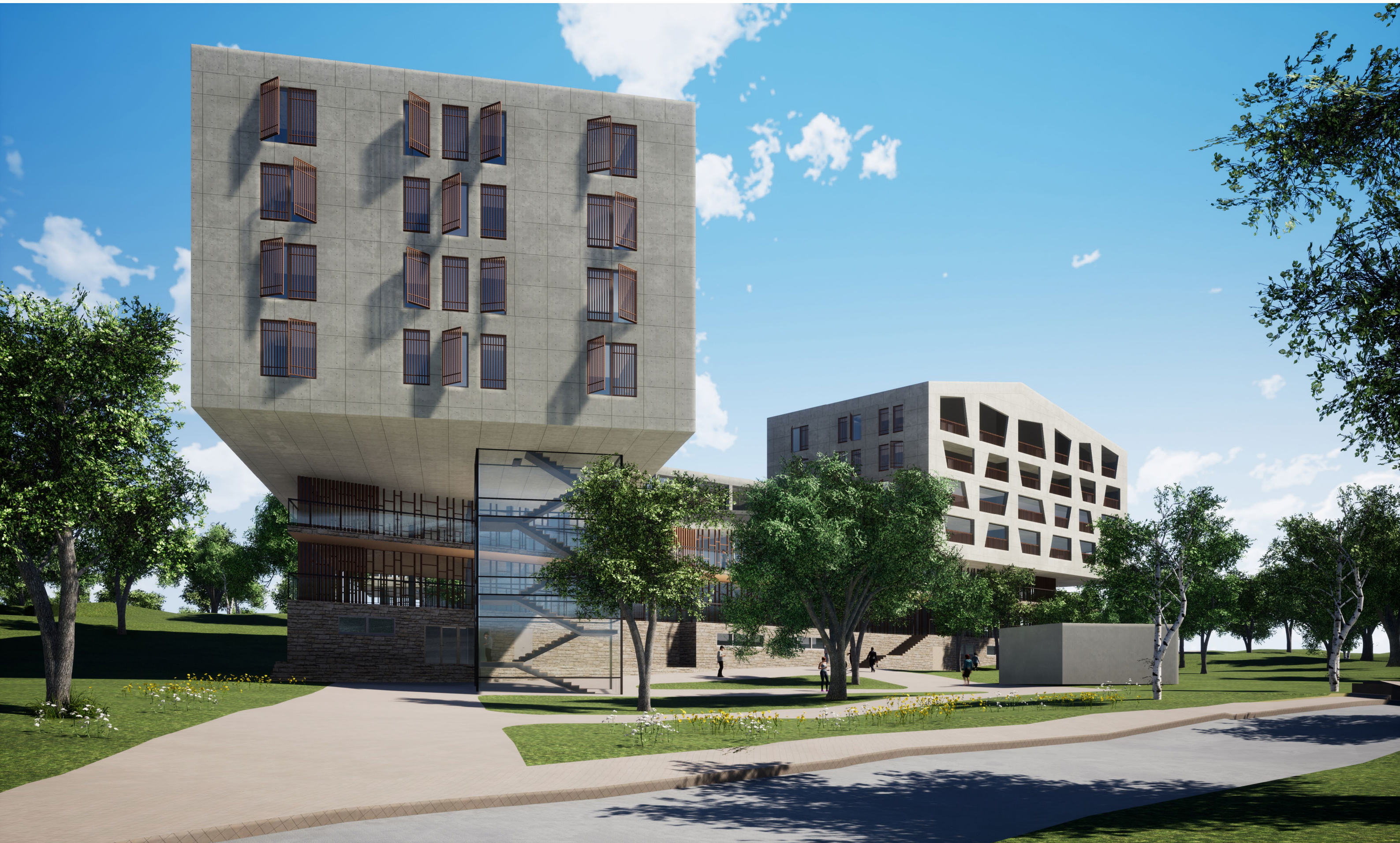
VIEW OF ENTRANCE OF UNDERGROUND FLOOR
