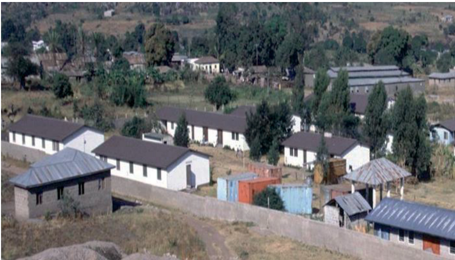
Figure 4. The buildings of the VET case researched, MHCC, in the early 1990s (Pylvänäinen 1991)
