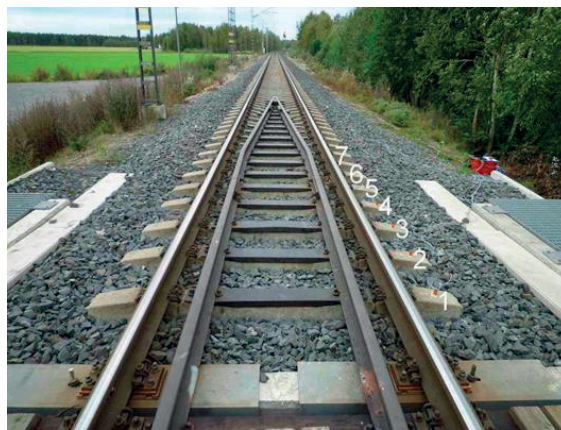
Figure 3.4. An example of using acceleration sensors to take measurements of recoverable settlement of a sleeper. The sensors are located outside the rails at the ends of the sleepers.
