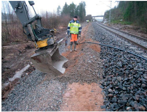
Figure 3.34. The settlement pipe being installed.
