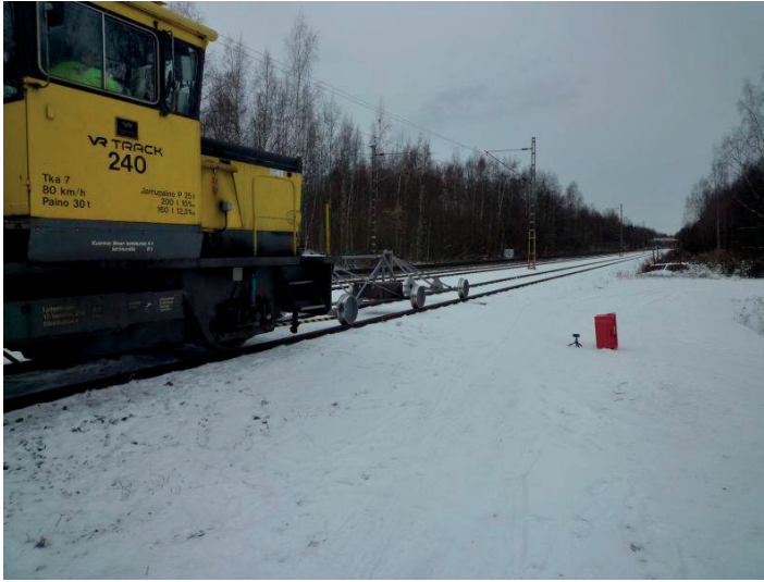
Figure 4.5. Calibrating the measuring device with a video camera. For this measurement, the device was calibrated by filming the deflection caused by a heavy axle at a known point in the track.
