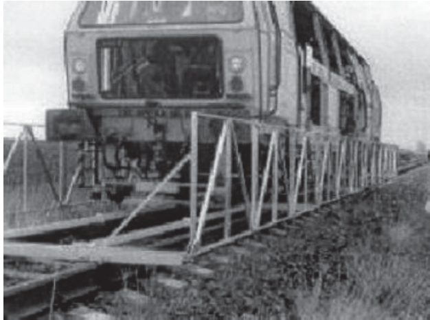
Figure 2.28. SKMT, the Czech measurement device (Berggren 2005).
