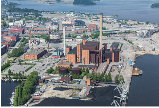
Figure 3.1: Hanasaari CHP power plant situated in Helsinki, Finland. The measurements in papers I, II and III were conducted at this power plant.
