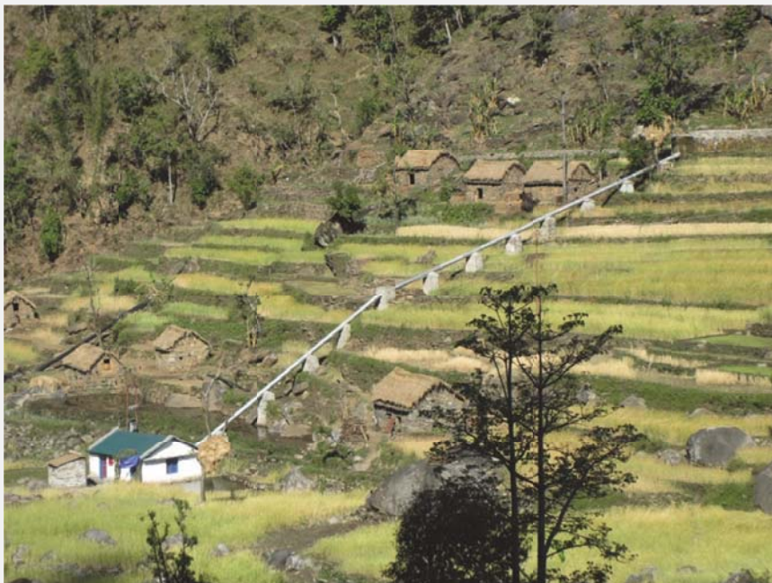
Photo credit: Bhatakatiya micro-hydropower plant and penstock pipe
