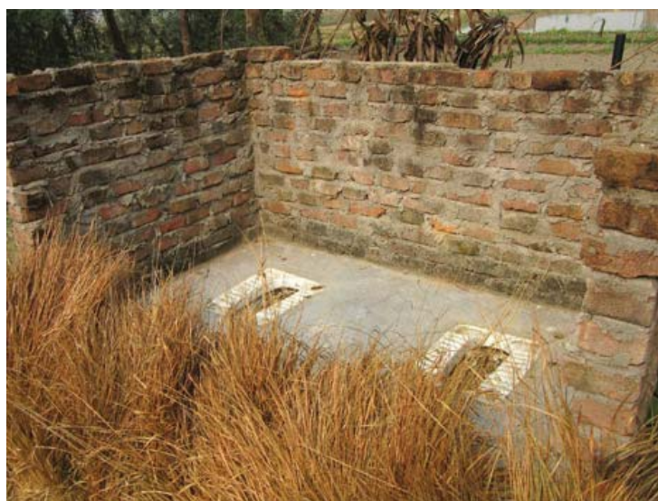
Photo 3 Subsidies remove the incentive for households to invest their own funds in a toilet and appear to change the way people think about toilets. Above, a subsidized double toilet with a half-completed superstructure. The household was waiting for an additional subsidy to finish the toilet.
