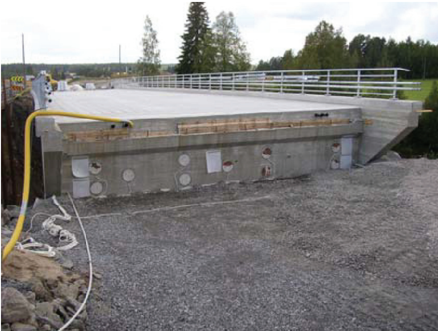
Figure 4.10 Installation of abutment earth pressure cells prior to approach fill construction.
