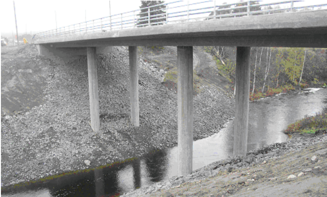
Figure 4.3 Haavistonjoki Bridge immediately after construction.
