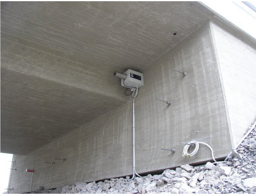
Figure 4.11 Laser distance-meter on the inner surface of the abutment.
