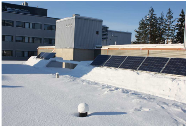
Figure 3.1: Example of partial shading of a PV string due to a building structure on a sunny day in spring 2012.
