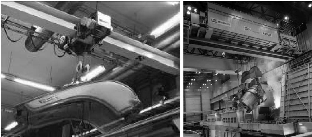
Figure 2.7 Two products with identical basic need and transformation process, vertical lifting and horizontal moving of goods. Assembly line (left), steel mill (right) (Konecranes Plc 2008).
