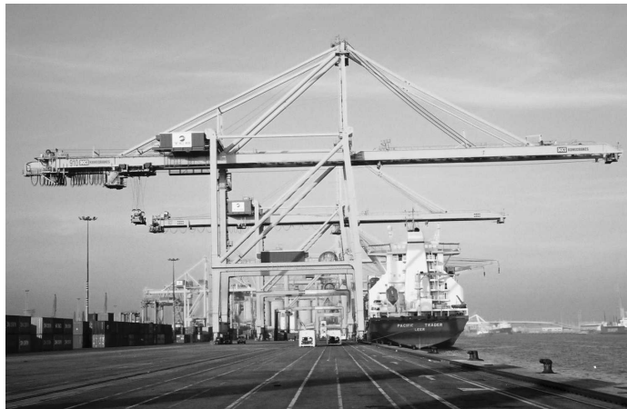
Figure 8.3 A ship-to-shore container crane used for loading and unloading containers from/to a vessel. Static concept has variations and is tailored to meet customer specific dimensions and characteristic (Konecranes Plc).
