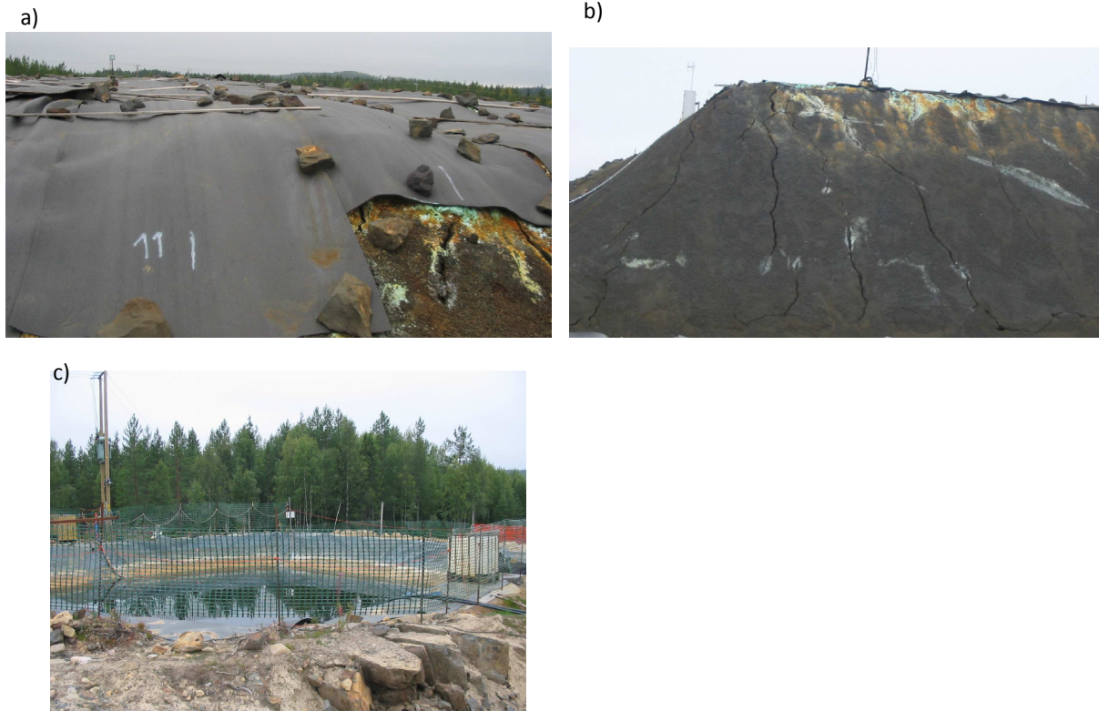
Figure 12. Photographs of demonstration-scale bioheap. a) Top of the heap covered with the plastic lining. b) Side view of the heap. c) Pond of the leach liquors. Photos: Kirsi Määttä.
