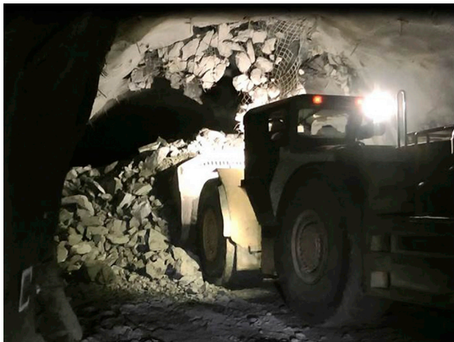
Fig. 4. CAT R2900G LHD working on typical size of rocks. For reference, the diameter of the LHD tires is about 2 m.
