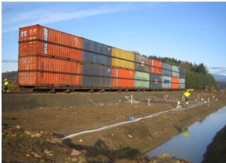
Fig. 6.1: Test site and containers before loading (Lehtonen et al. 2015).
