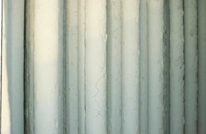
Fig. 1.1: Fume deposits in the boiler bank (courtesy of H. Tran).
