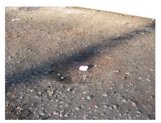
*Fig 5.1. A hole caused by fuel spillage on an asphalt forecourt pavement made of asphalt. Matchbox indicates scale.*
